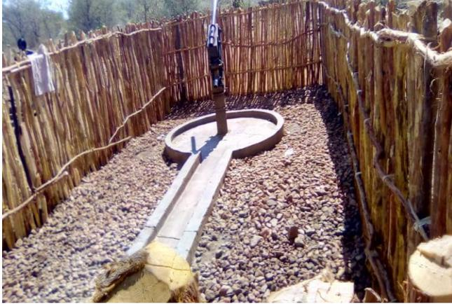
*Figure 2: One of the 59 boreholes assessed for rehabilitation in Jaji 2 Village. The borehole requires rods, GI pipes and a soak away pit.*
