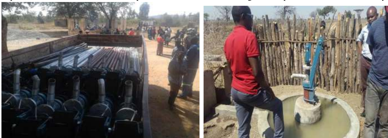
Fig1 & 2 Show WP spares and fitting of a Pump Stand Unit
