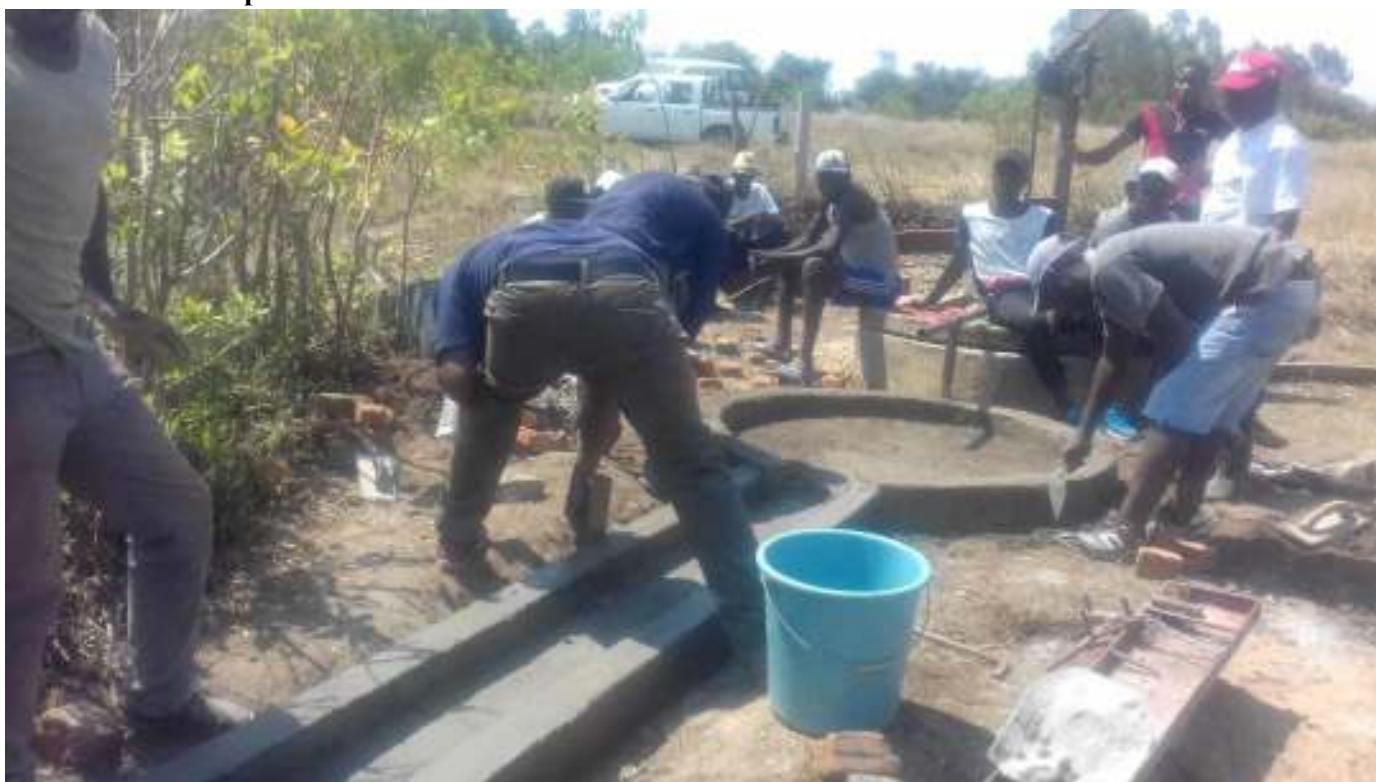
Fig 3 Apron builders putting finishing work to Deep Well
